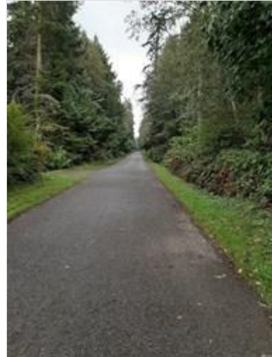
View looking south on N Bay Way, lot on the right.
