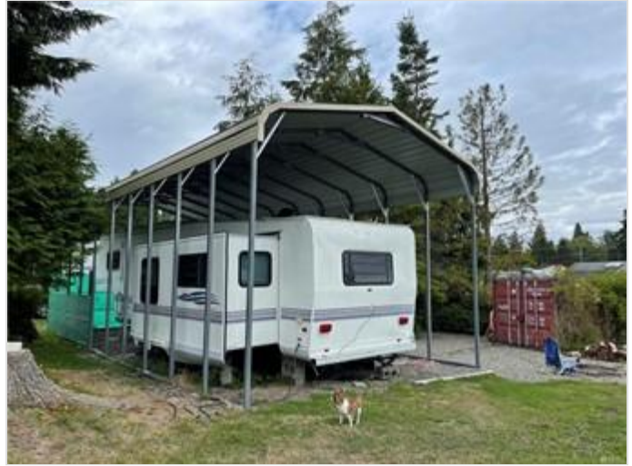
Metal carport to protect the larger RV
